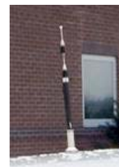
5 dBi 2.4 GHz Antenna
