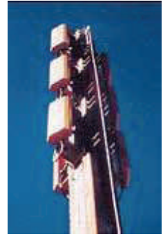
3 Carrier Laminated Wood Structure
